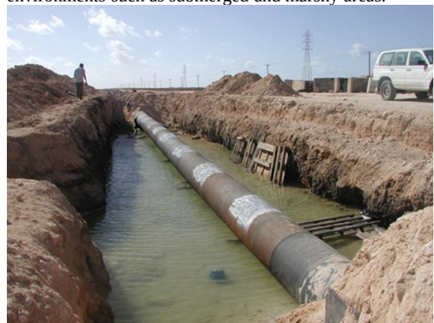
Figure 17: Immersed Pipeline Below sea level (sebkha area) [2].
