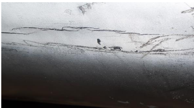
Figure 3: External Axial Stress Corrosion Cracking, determined by Rosen Smart Pig [1] [2]
