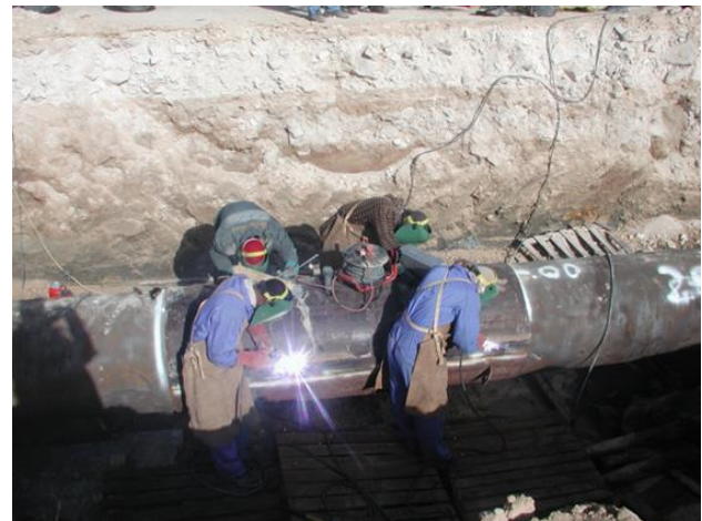
Figure 6-Welding Technique considering the cooling time [1].
