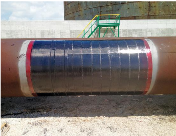
Figures 11: Composite Wrap Repair for Non- Leaking defects [3].
