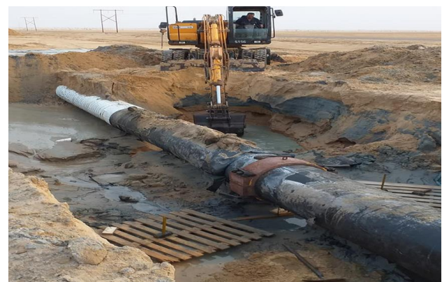
Figure 8- Installation of Split Repair Clamp and Bolted up & Torqued [1].
