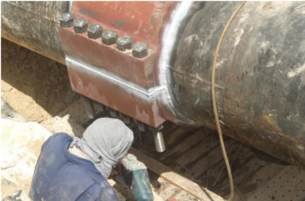
Figure 9- Converted the Temporary Clamp into Permanent by welding [1] [2].
