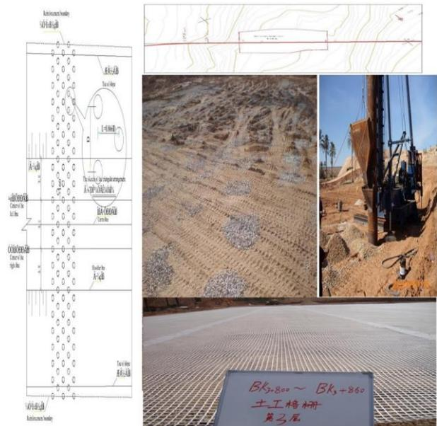
Figure 6. Crushed stone pile and geogrid in pilot section
