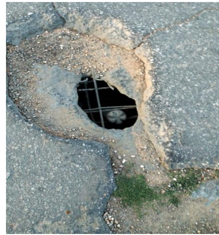
Figure 8. Explosion holes
