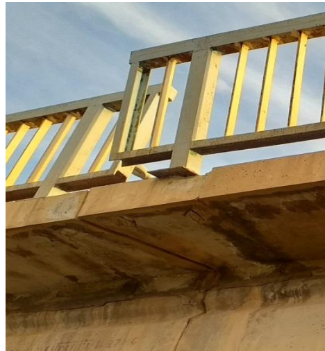
Figure 15. Iron fence slope.
