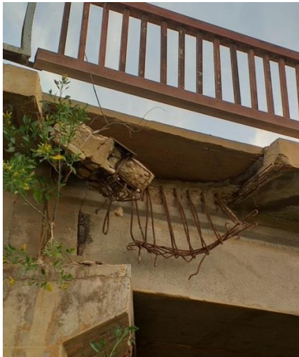
Figure 14. Sidewalk explosion.
